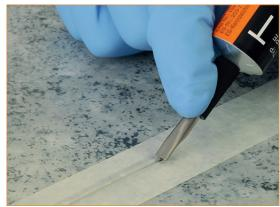
After about 60 minutes pull off the masking tape backwards at an angle.
