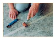
Press the special masking tape firmly to the PVC-floor covering by using a seam roll.
