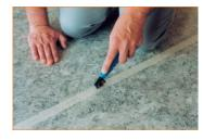
Easily cut the masking tape with the rolling knife in the seam area. Alternatively a straight blade can be used.
